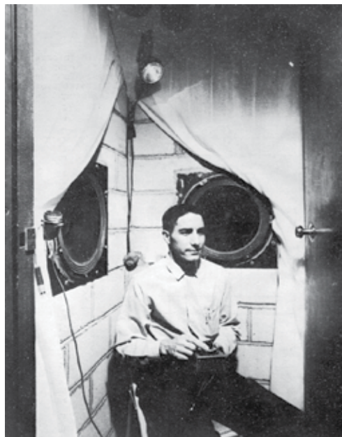
Figure 9.109. BBN Sonic Boom Test Chamber with curtains drawn to show low frequency speakers (ref. 9.61).
